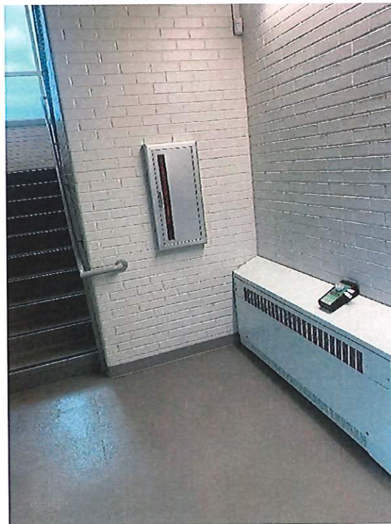
Figure 10. Location of Air Sample A12 – Stair W1
