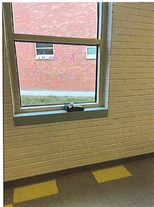
Figure 29. Green Wing Hallway and location of clearance sample A4. Figure from re-test taken on November 7, 2023.
